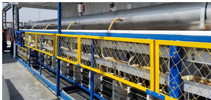
Demonstration Unit Installed in Peru
