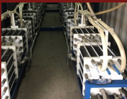
Electrolysis Cell Stacks
