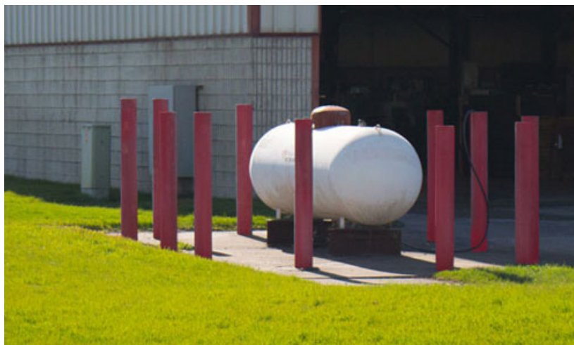
Figure 2: Bollards protecting a compressed gas storage tank from potential vehicular damage [10]
